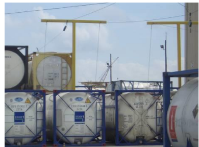
Figure 8.12 Fall arrest stanchions
